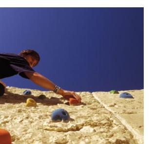
This very long and organically shaped climbing wall in Munich also serves as an embankment. It shows that even a demanding piece of sports equipment and playground element can be created from a simple retaining wall.
